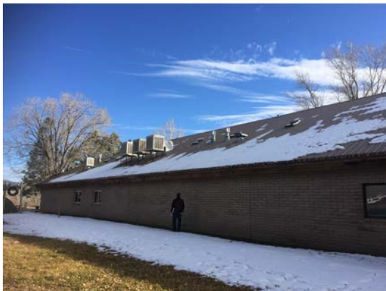
Photo 3: Roof mounted evaporative coolers
