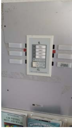
Photo 5: existing, unused fire alarm panel at entry
