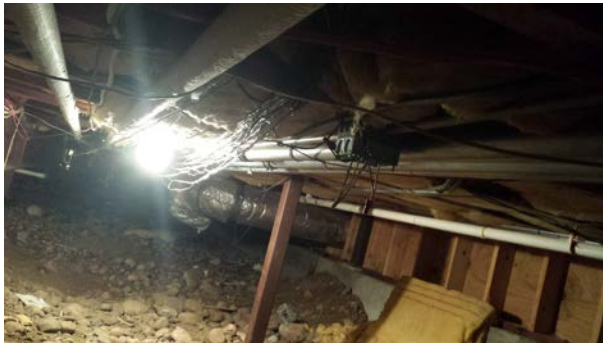
Photo 7: Unsupported crawl space cabling, open j-boxes
