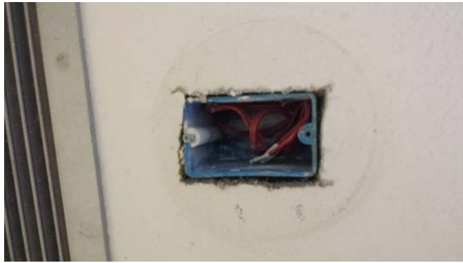
Photo 6: Missing fire alarm device
