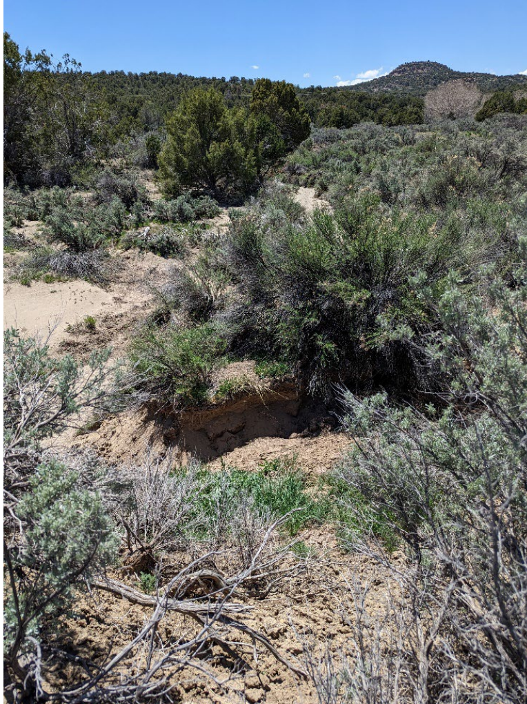
Photo 9. Looking upstream at Cottonwood Canyon drainage crossing 9a.
